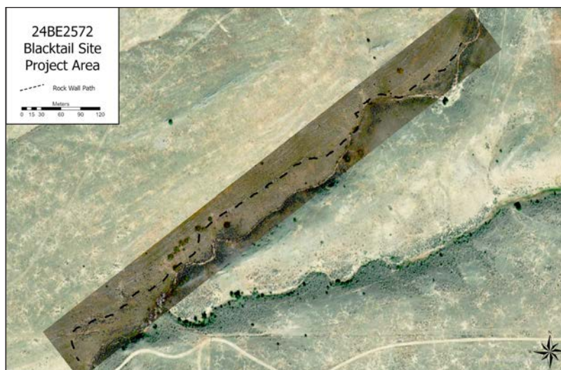
Figure 2. Aerial view of the Blacktail drift wall site. The dark dashed line shows the wall’s location above the northeast branch of Cabin Creek. The wall terminates in the creek bottom.
