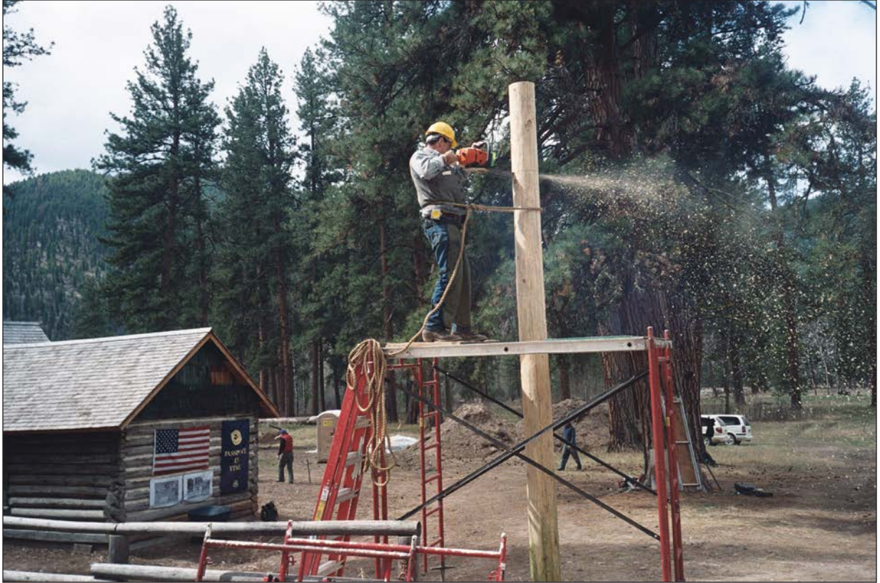
Figure 13. Gene Thompson installing an entryway post at Morgan-Case.
