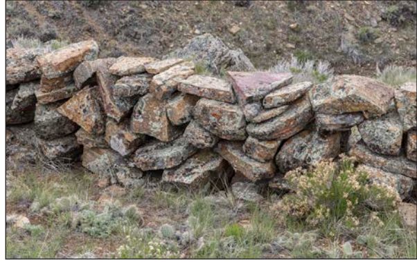
Figure 5. Detail of the four-to-five-courses of granite gneiss rock wall at the Blacktail site. Note that the lowest rocks are embedded in soil and vegetation, and all rocks are lichen-covered.
