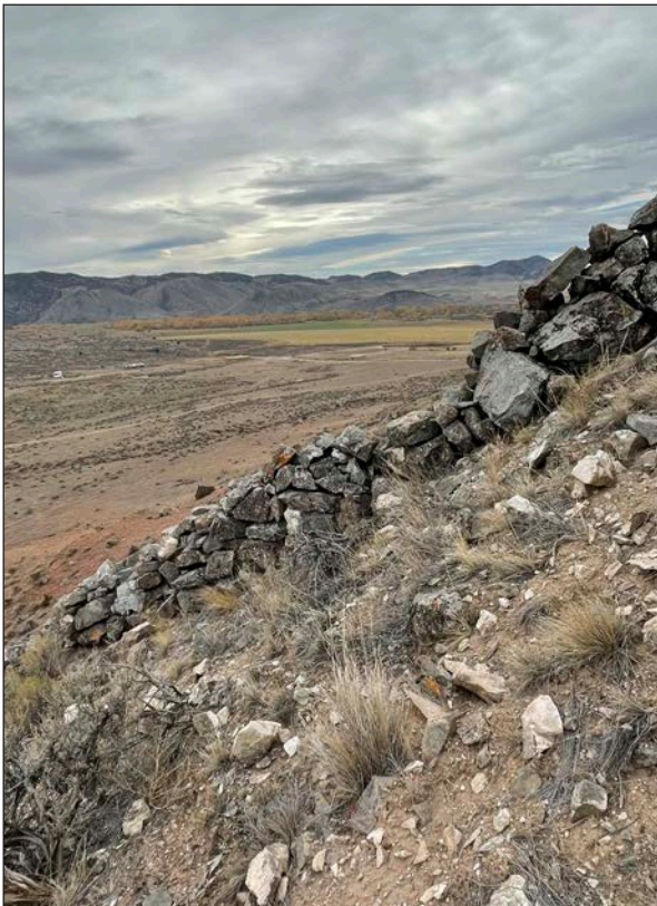
Figure 11. Closeup of the rock wall descending into Creasey Gulch. The wall is comprised of 4-5 tiers of stacked rock obtained from the abundant rock outcrops on the steep slope.
