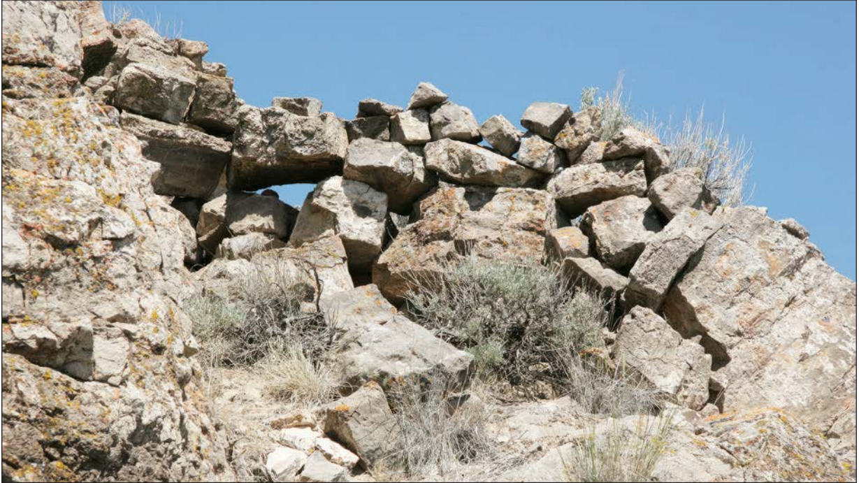
Figure 12. Closeup of Creasey Gulch descending rock wall showing the careful stacking of rocks to increase wall height.
